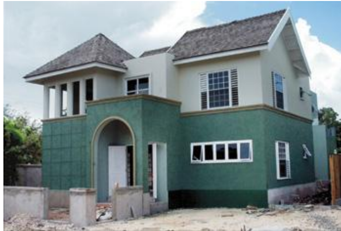
One of the units in the complex. (Photos: Bryan Cummings)
